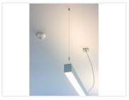
Motion sensor with a built-in light sensor, so the sensor only switches on, when it is dark in the room. It saves power by not turning on the light when it is not unnecessary.
